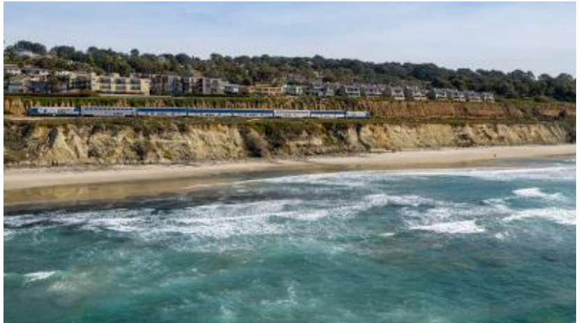
The LOSSAN Agency Board of Directors provides oversight of key initiatives outlined in LOSSAN Agency's annual business plan including management of the Amtrak Pacific Surfliner service.
